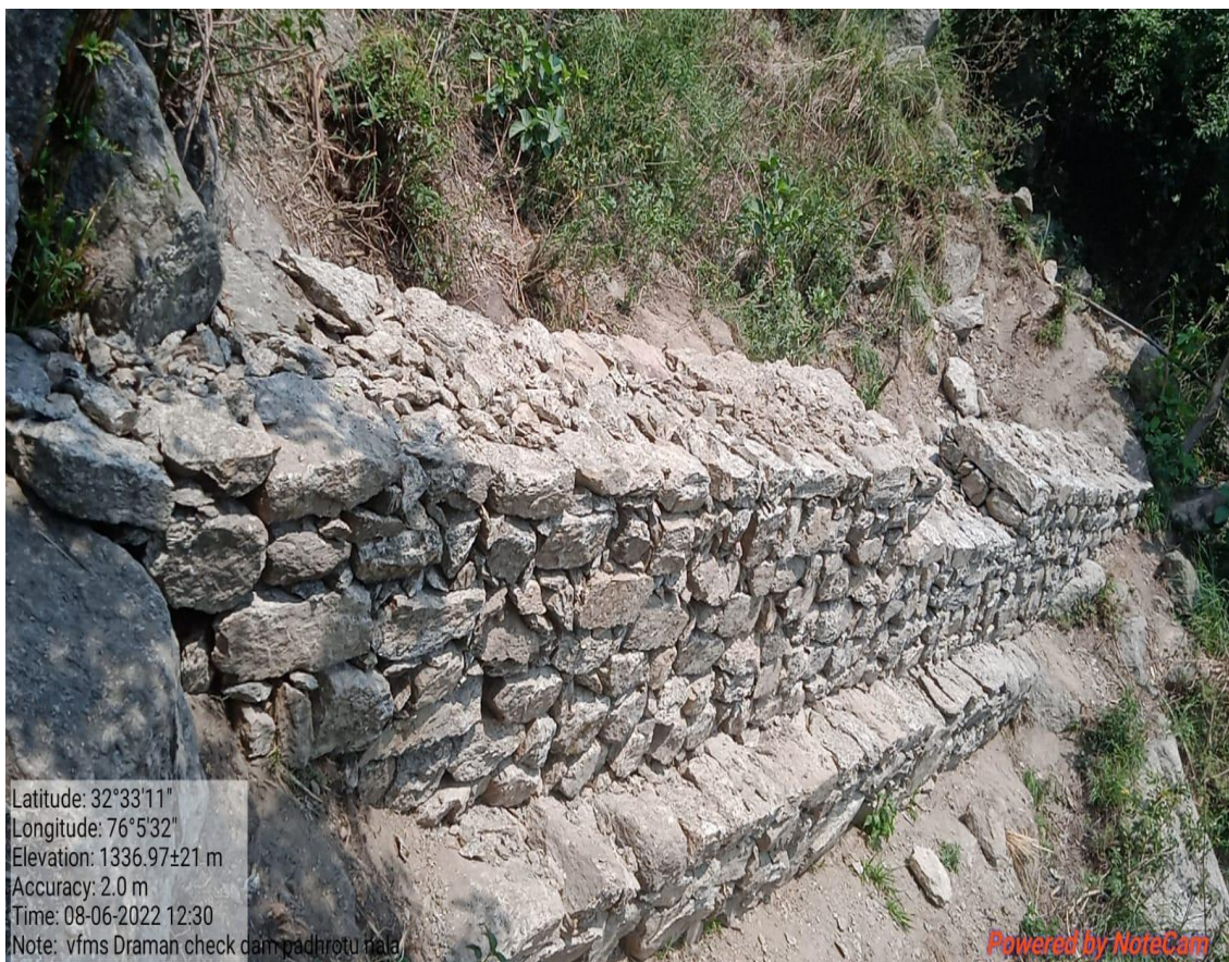
Dry stone check dams at VFMS Draman(2022-23)
